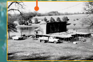
Small Lakes stage being constructed.
